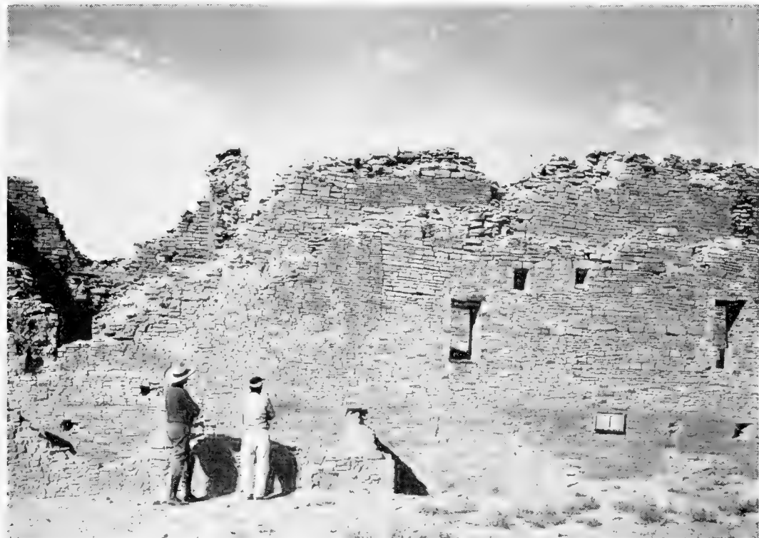
FIG. 166.—Outer south wall of Pueblo del Arroyo, showing varied stonework and later, abutting rooms. (Photograph by Neil M. Judd. Courtesy of the National Geographic Society.)
